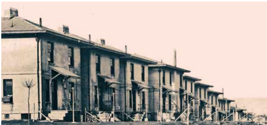
Prairie style housing c.1917 built with Edison technique at Cement City in Donora, PA. Photo: Donora Historical Society.
