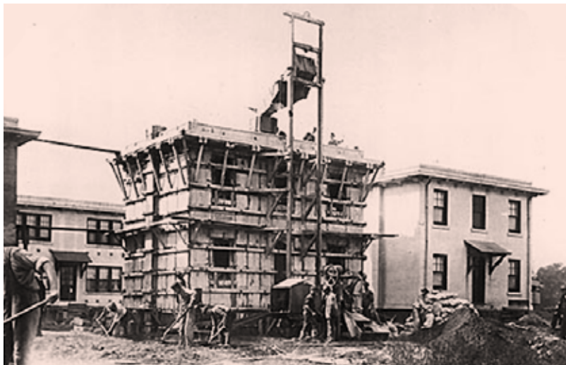
Edison house casting showing single pour in process on rooftop.
