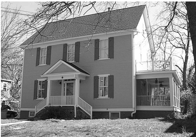
7321 Takoma Ave. beautifully restored and saved for posterity.
