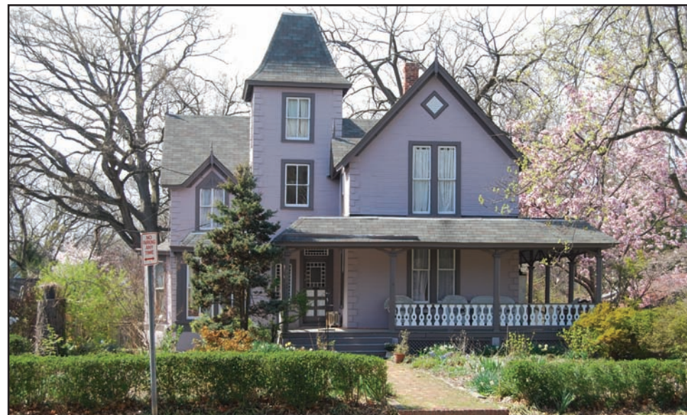
Completed in 1885, the Bliss House on Maple exemplifies the elegant living Gilbert proclaimed in his brochures.
