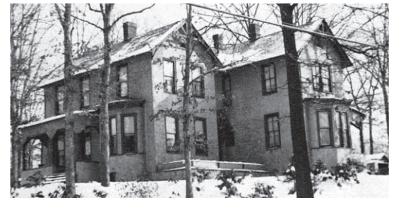
As part of the addition, the clapboard siding was replaced by stucco. The house survived demolition threats and continues to offer a glimpse of life in early Takoma Park.
