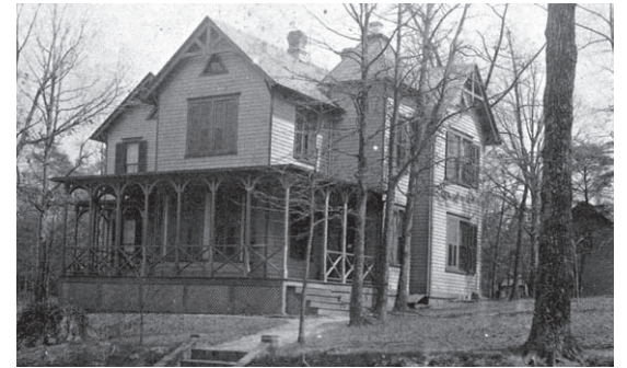
The house as it first looked before the 1890 addition. The sense of being hidden in the woods remains a feature today.
